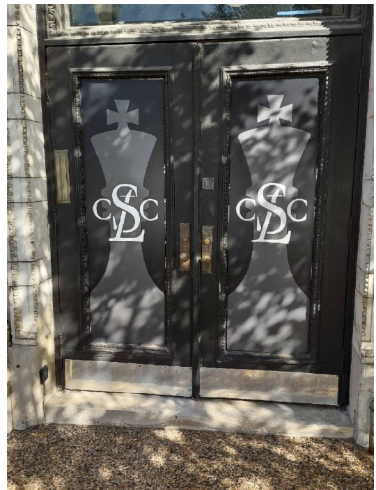
I did not enter through these doors because of the renovation, but instead another door at the other end of the building.
